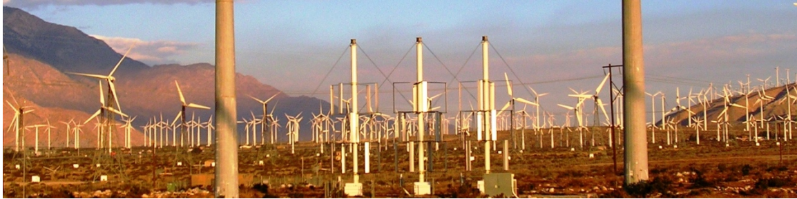
Three Windstar 530G VAWTs among HAWTs in the San Geronio Wind Resource Area , California
